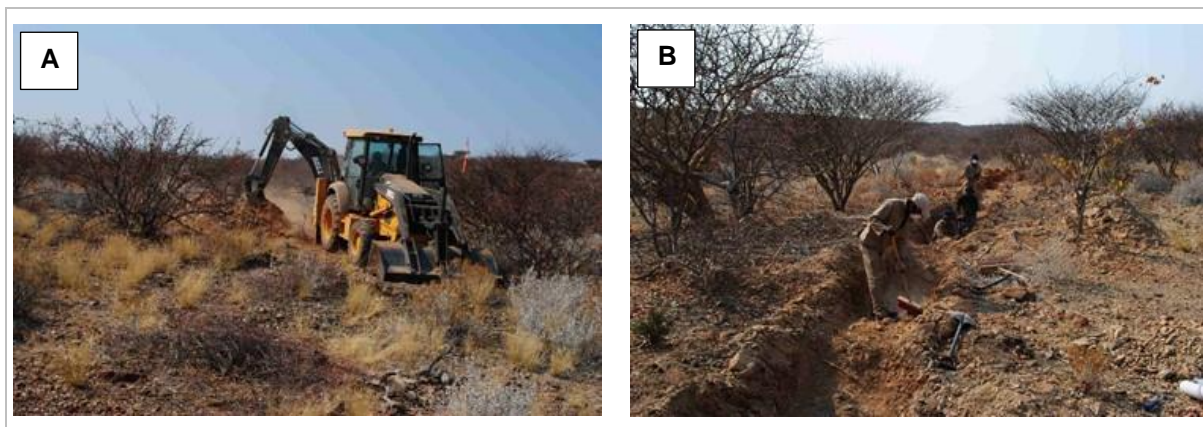
Figure 9-5 A – Digging Trenches on Area 2B with a Backhoe, B – Cleaning Trenches in Preparation for Sampling and Mapping
