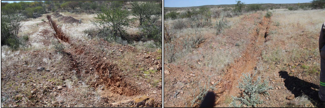
Photo 5. Typical N-S transverse exploration trenches through starter pit, area 4.
