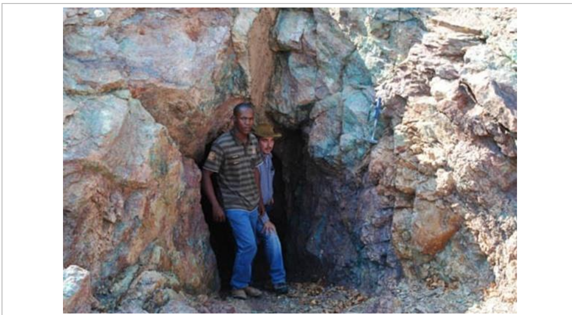
Figure 6-1 Adit at the Former Lofdal Copper Mine with Copper Staining Around the Portal
