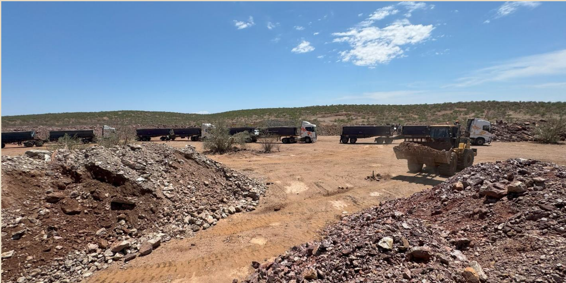
Loading of the first truck fleet with Block 1 material
